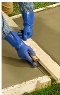
11 ■ Cut control joints in the concrete after the concrete sets up
