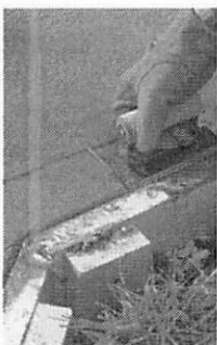
10 ■ Shape the edges of the concrete by running an edger along
